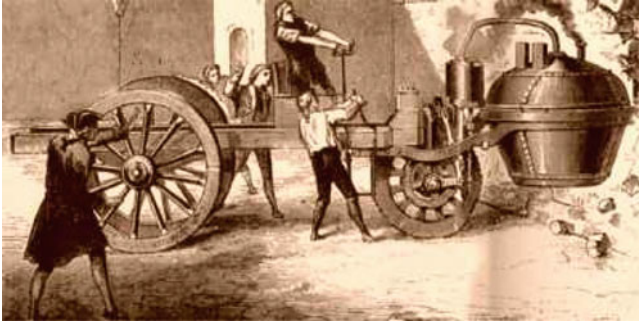
Fig. 3.4 1771 crash of Nicolas Joseph Cugnot's steam-powered car into a stonewall. Cugnot was the inventor of the very first self-propelled road vehicle, and in fact he was also the first person to get into a motor vehicle accident
